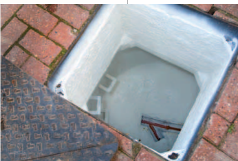
Manhole sprayed with Ultracoat
